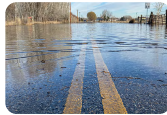
Surface Water Flooding
