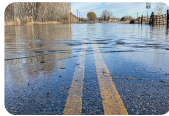
Surface Water Flooding
