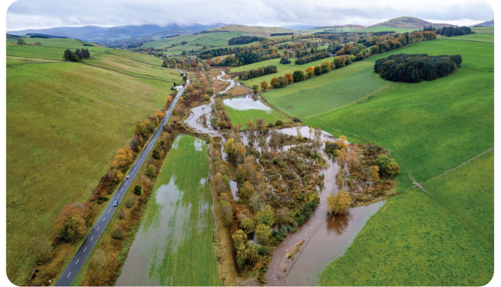
Eddleston Water after Natural Flood Management
